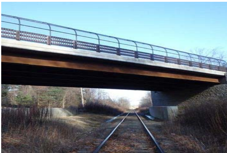
The Massachusetts DOT used GRS-IBS to build a bridge over a rail line.
