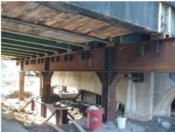
Figure 2. Span 9 shoring via steel moment frames.
