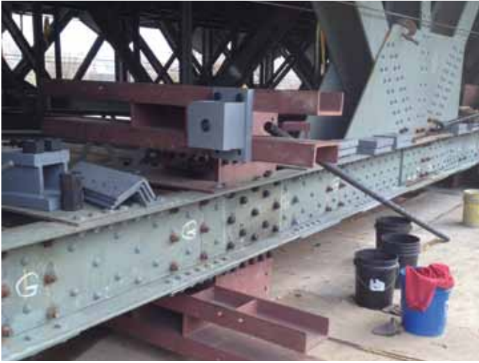
Figure 7. Transfer plates and channels.
