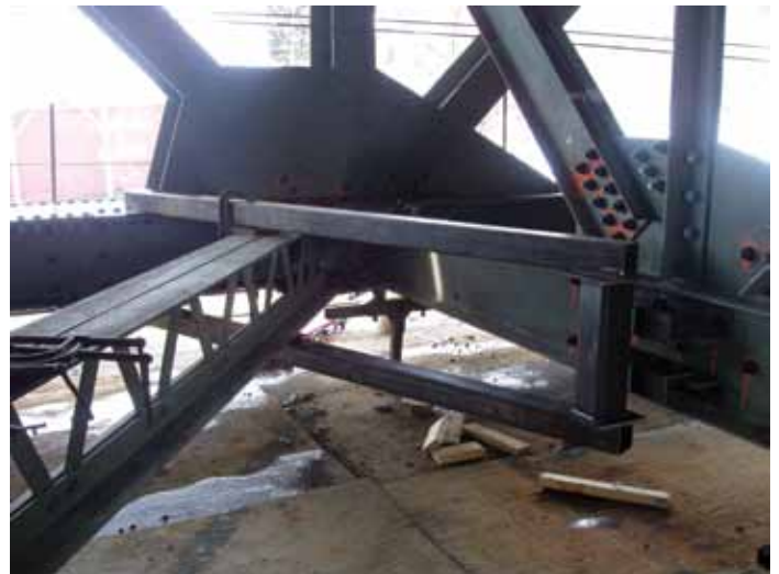
Figure 3. Bottom lateral retrofit shoring.
