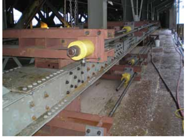
Figure 8. Hydraulic rams and threaded rods.
