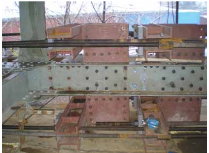
Figure 6. Vertical transfer plate as constructed.
