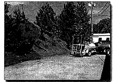
Figure 5. Hydroseeding the slope
