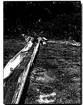
Figure 21. Split pipe with soft matting
