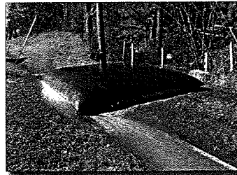
Figure 34. Sediment bag and its treatment ditch
