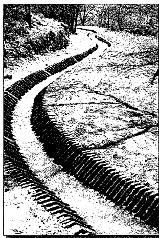
Figure 18. In-ground treatment ditch
