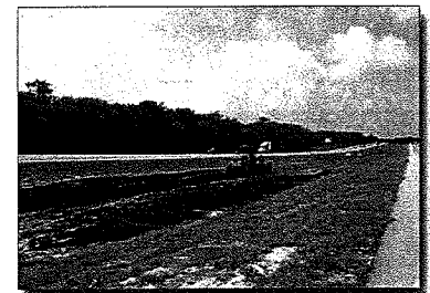
Figure 37. Recycling sediment along a highway
