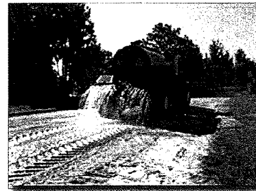
Figure 11. Water truck applying dissolved polymer flocculant
