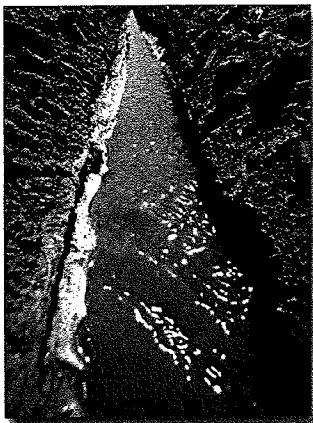
Figure 23. Untreated furrow with erosion
